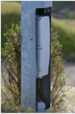
Inside of tower
