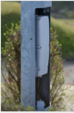
Inside of tower
