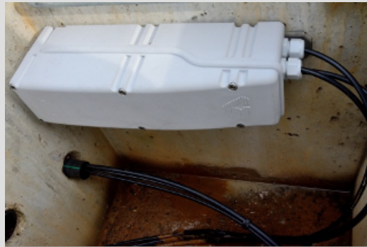
Installation in cable chamber (LIT)
